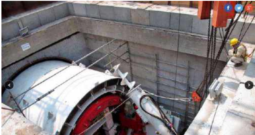
Gambar 2.10 Perakitan TBM di Launching Shaft
