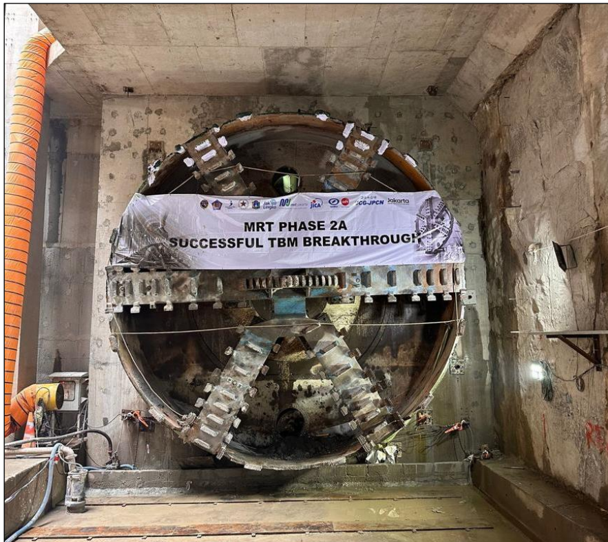
Gambar TBM 1 Breakthrough Northbound Tunnel di sisi utara Stasiun Bundaran HI
